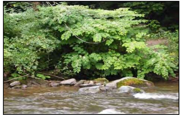
In this photo, the rocks protect the knotweed infested bank from the main current, which should both slow the water and any associated erosion. Nevertheless, there is a large hole underneath this stand of knotweed, and bank erosion continues downstream of the knotweed until the edge of the photo.
