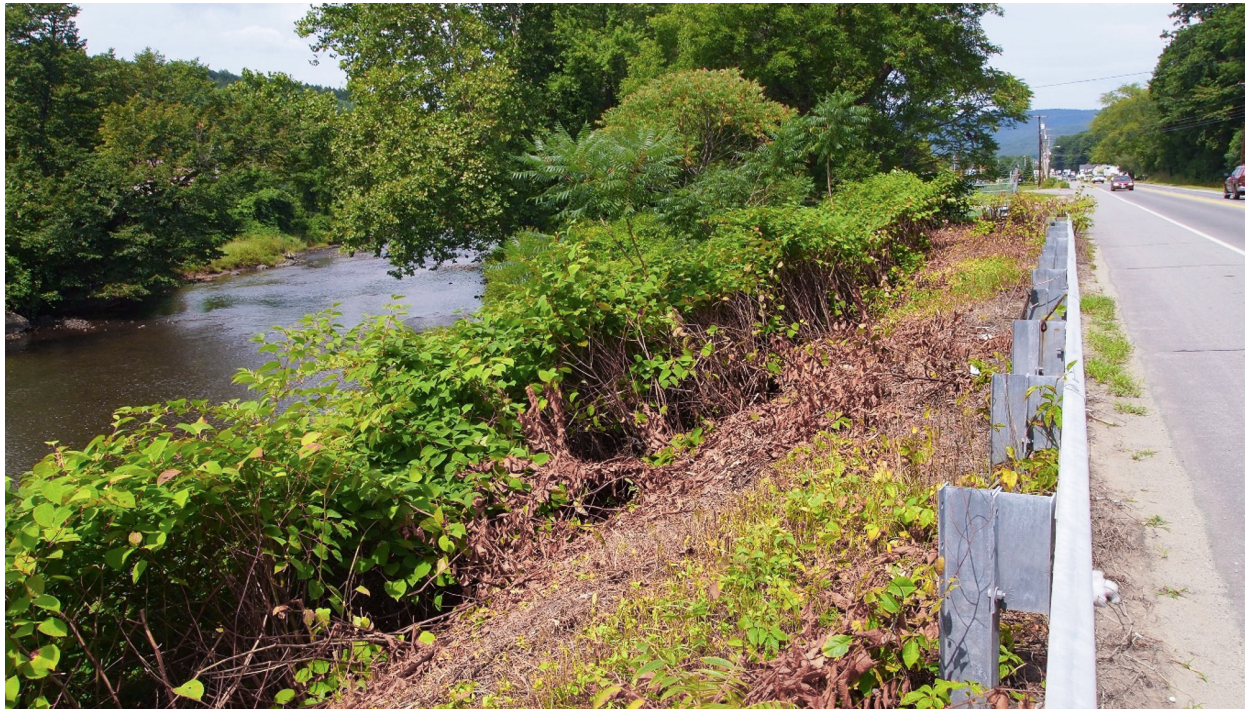
Black River Roadside: This knotweed along Vermont's Black River is being managed by mowing, which will spread the knotweed further, since pieces of knotweed can root and grow. Additionally, sudden failure of this bank during a storm would significantly impact the roadway.
